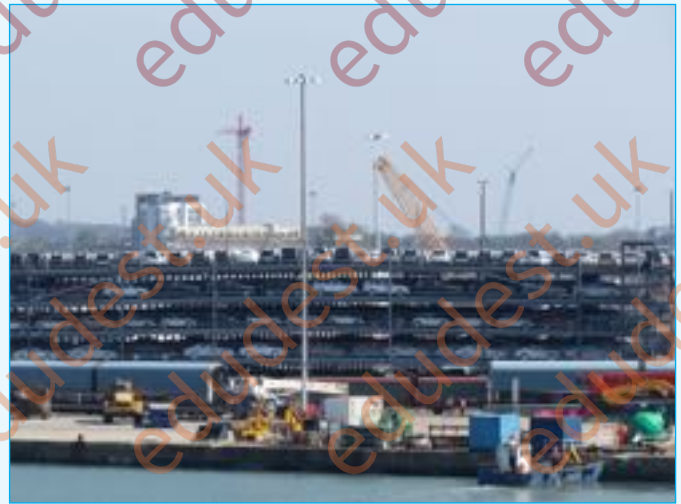
Image showing the multi-deck terminals in the eastern docks.
