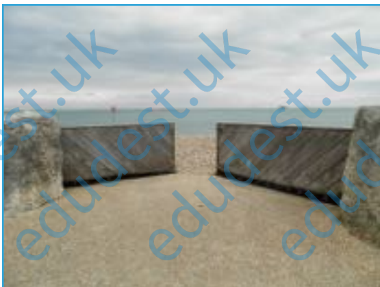
Limestone gate portals and heavy marine hardwood gates with stainless steel frames
